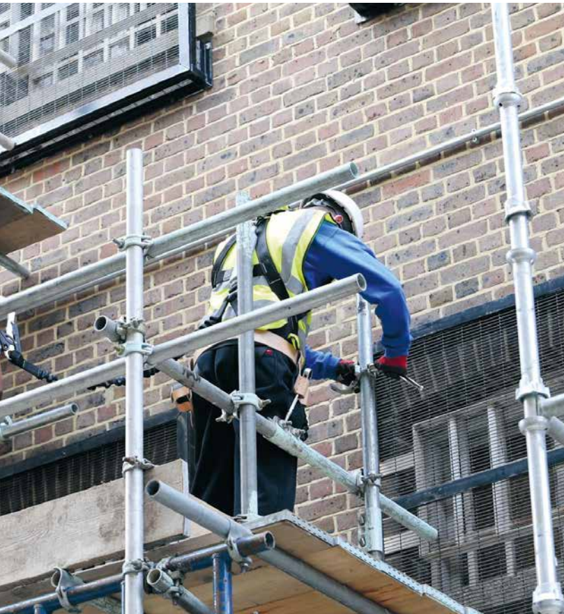
Trainees constructing a scaffold platform at our Academy at HMP Brixton
