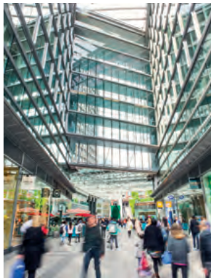
Cardinal Place, SW1 Landmark site, part of our Victoria cluster, home to blue-chip businesses and retailers. Annualised net rent £29.1m
