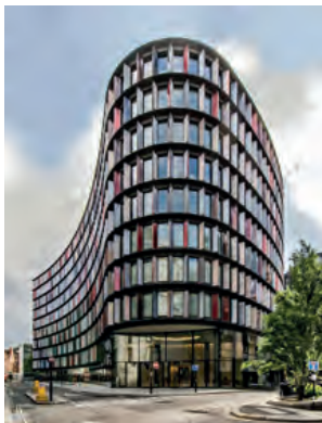
1&2 New Ludgate, EC4 Contemporary office, restaurant and retail space. Annualised net rent £22.3m
